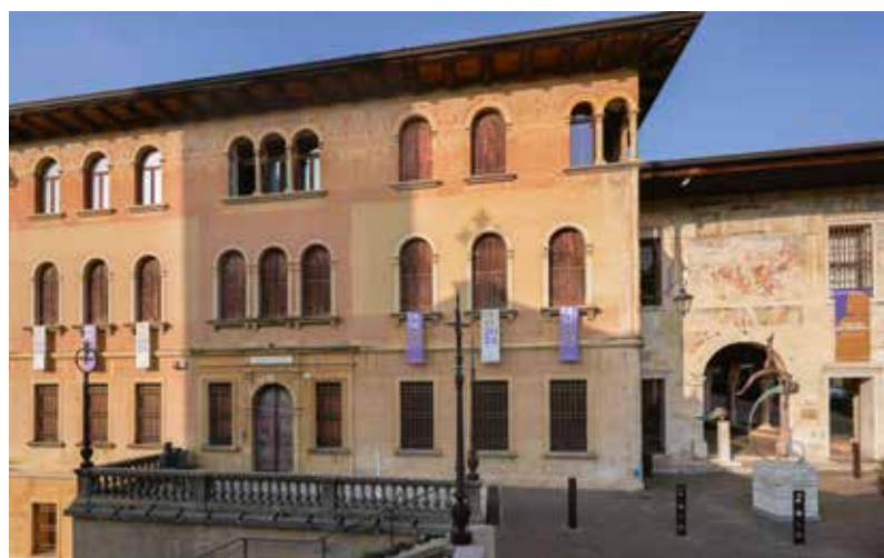
On the right: a view of Villa Cipriani in Asolo, courtesy the hotel
